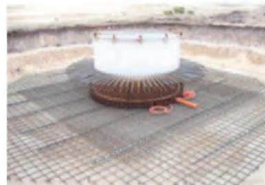
Figure 1 – Steel reinforcement being added to foundation
